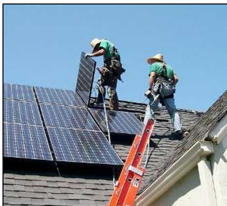
Fig 13. A green job is being able to install solar panels
