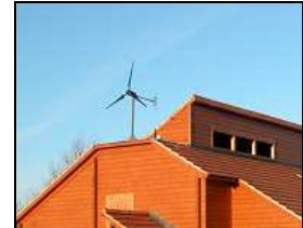
Fig 41. Wind turbine at Stonehaugh Community Hall. The placing must not be negatively affected by the vernacular design, as it was in this instance
