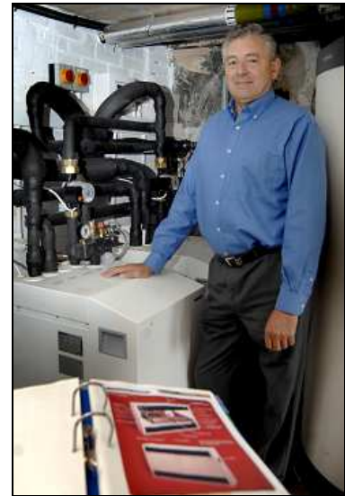
Fig 30. Geothermal heat-pump at Bellingham Town Hall
