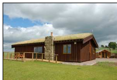
Fig 23. The Hytte at Bingfield has a grass roof. This provides insulation, helps to reduce rainwater run-off, and is also aesthetically pleasing. The holiday accommodation has a geothermal heat pump, and a Green Tourism Business Scheme Gold Award
