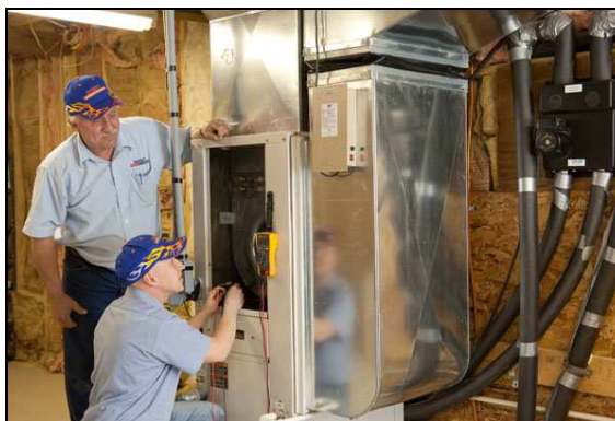
Fig 14. A green job is being qualified to install geothermal heating pipes
