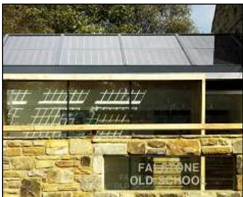
Fig 45. Falstone Old School Tea Rooms
