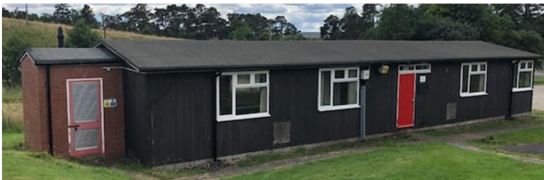
Figure 1 Example of an existing block (no. 95) to be demolished and replaced by the proposed development
